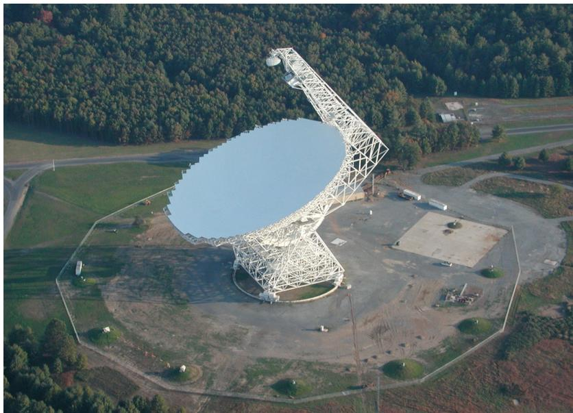
**Figure 2.1:** The Robert C. Byrd Green Bank telescope located in West Virginia, USA. It is the largest steerable radio telescope in the world, with the reflecting dish having a diameter of 100 m. The telescope can operate at frequencies ranging from 290 MHz to 116 GHz using receivers which are sensitive to different frequency ranges. The off-axis support arm houses these receivers. Image credit: National Radio Astronomy Observatory.
