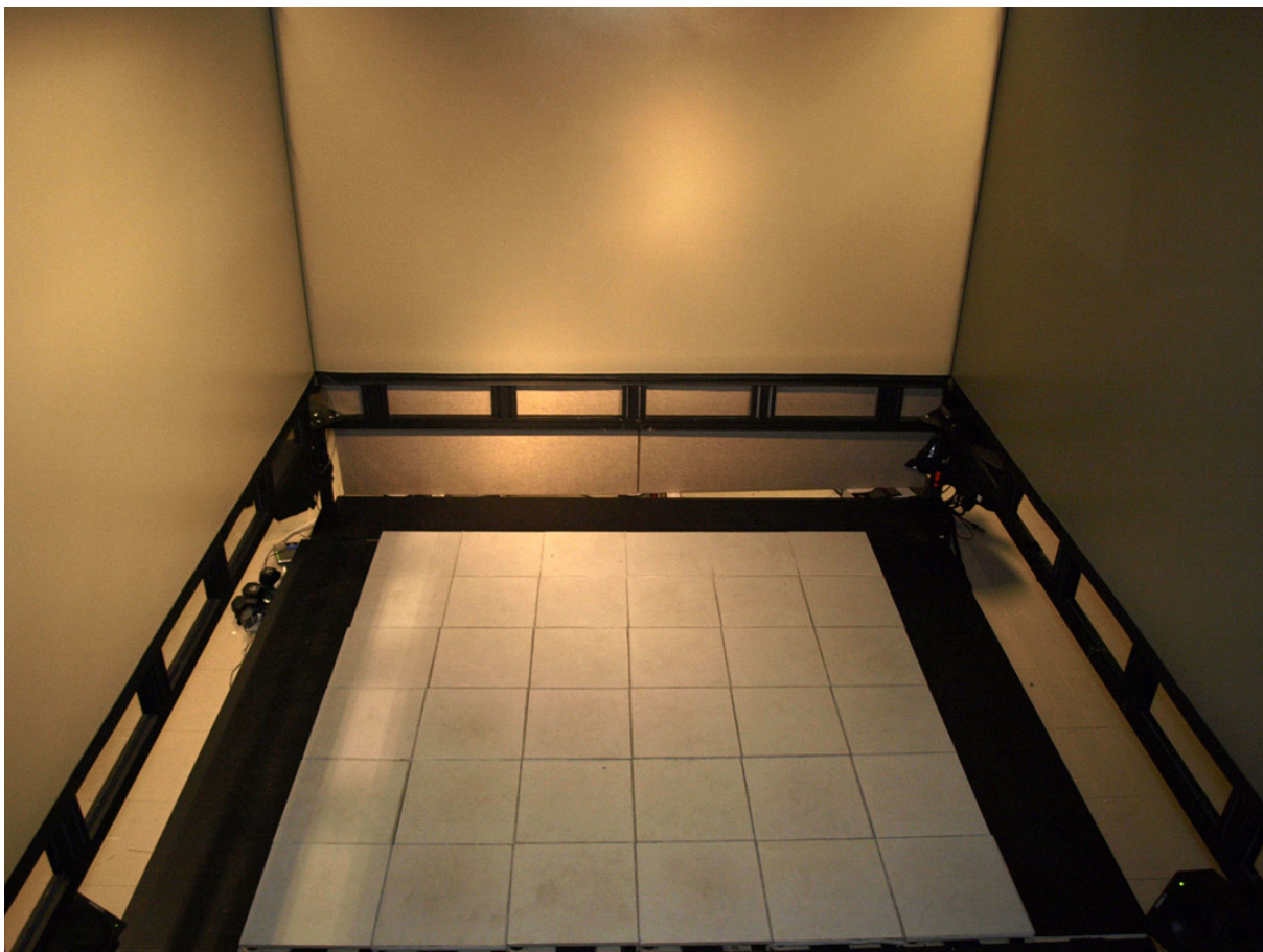
Figure 2.18 The completed floor inside the lab's CAVE.
