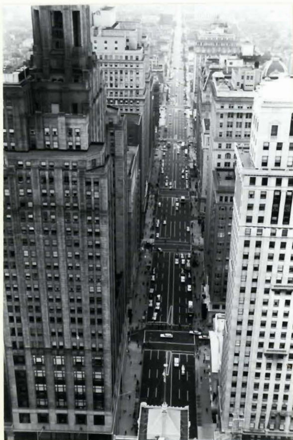
BROAD STREET LOOKING SOUTH FROM CITY HALL TOWER
