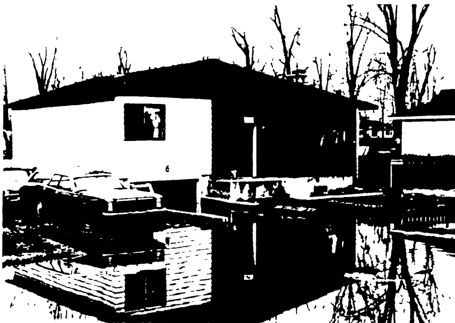
Photo. 5.3c In comparison to previous picture residential dwelling is unprotected by infilling measures (spring flood 1984)
