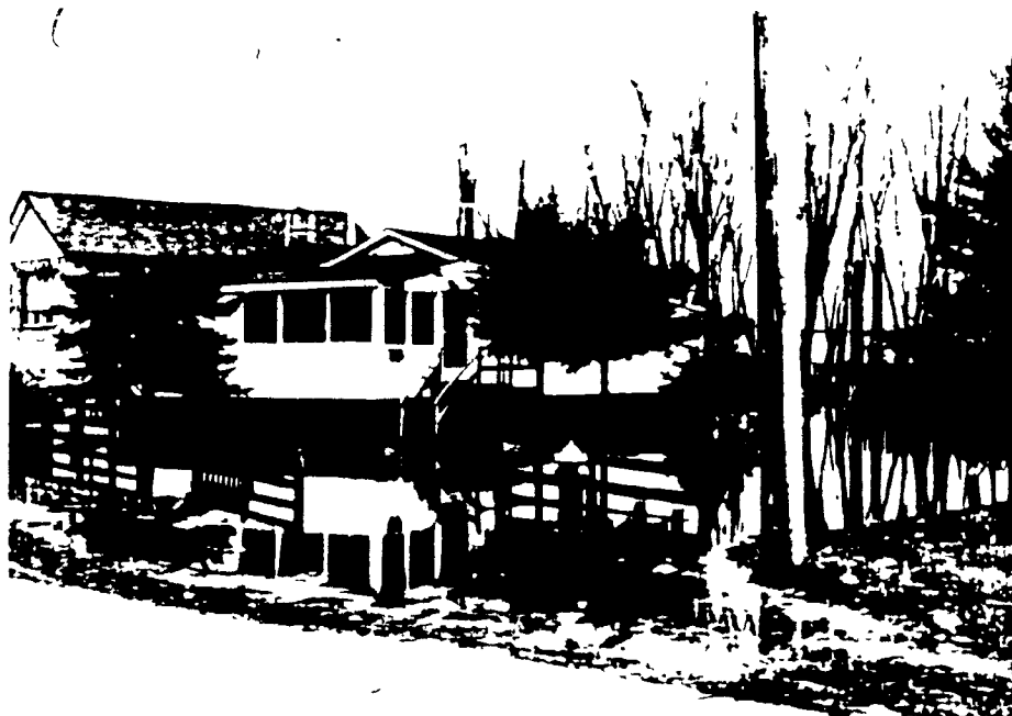
Photo. 5.3d Cottage converted into a permanent residential dwelling - the structure has retained the cottage's "stilts" as adaptation to floodplain environments which is less disturbing than infilling.
