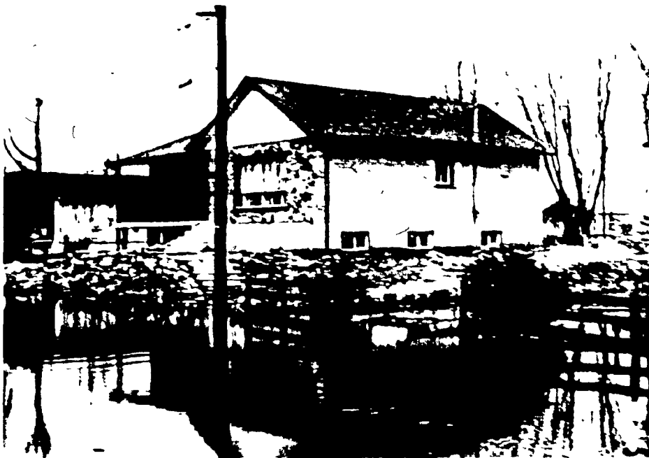
Photo. 5.3b Example of recently constructed dwelling raised above flood heights by infilling (1984 spring flood).
