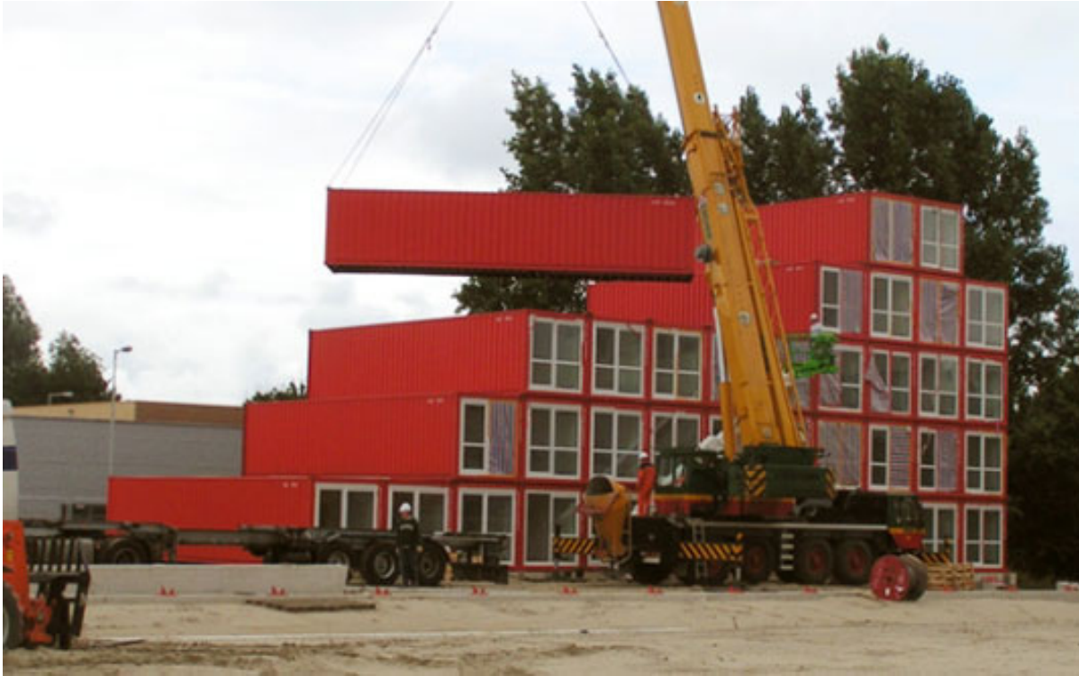
Figure 4 - An example of modular building using repurposed shipping containers. http://inhabitat.com/prefab-friday-keetwonen-container-student-housing/wp-content/blogs.dir/1/files/keetwonen2.jpg
