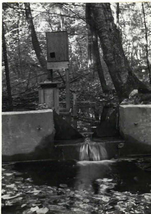
Illustration 8. View from downstream side of weir and stream gauge.
